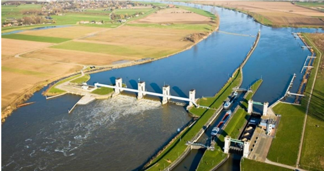
Figure 7. Damming at Lith (Meuse). On the left the hydropower plant and fish pass, on the right shipping sluice (photo: Rijkswaterstaat).
